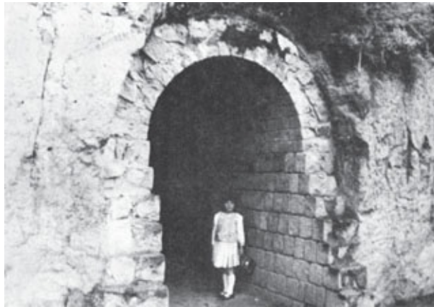
Fig. 10.4. La Olla . Outside entrance of tunnel. Facing stones have been removed.
