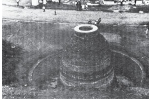
Fig. 10.3. La Olla or The Oven. Strange building from prehistory recently uncovered on the top of Panecillo. This dome has no architectural counterparts in the entire world, except for the mysterious melted wall "Scottish Ovens" with circular openings in their tops.
