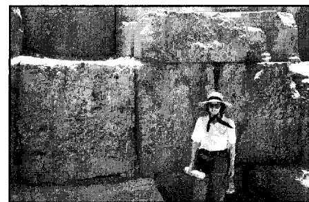
Outer stones of the Great Pyramid showing close fit of stones and little mortar. Source—G. Little.
