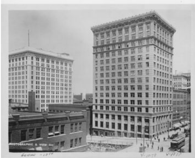
R.A. Long Building – James J. Lynn’s company office – 928 Grand Ave., Kansas City, MO (northwest corner of Tenth and Grand Avenue).
