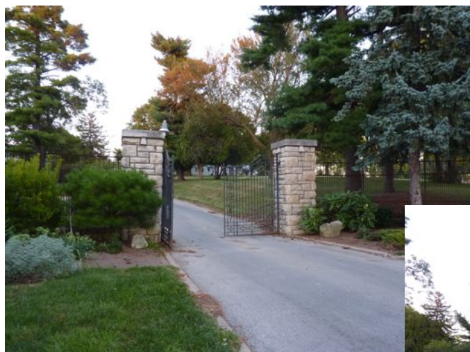
Front gate and fence.
