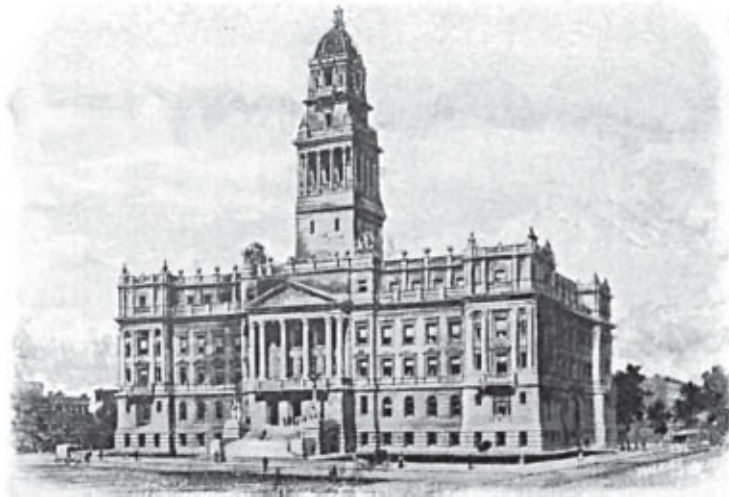
The Wayne County Building in Detroit where the Cayces most likely went to trial.
